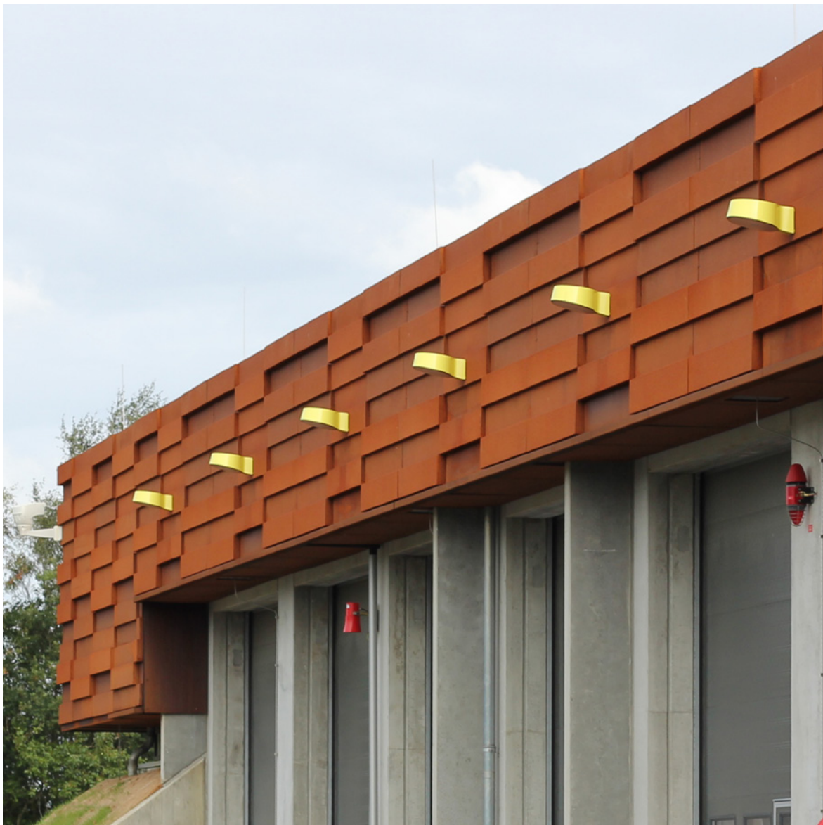
Egtved Gas Compressor Station, architects: C.F. Møller
